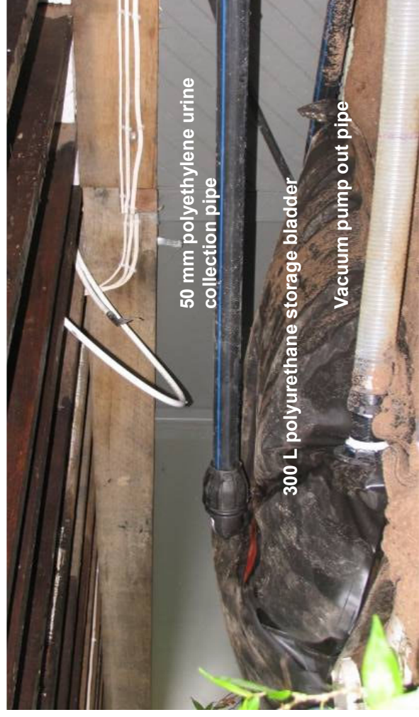
Figure A. The 300 L urine storage bladder (full) under the residence showing the urine collection pipe and the reinforced vacuum pumpout hose for emptying the bladder.
